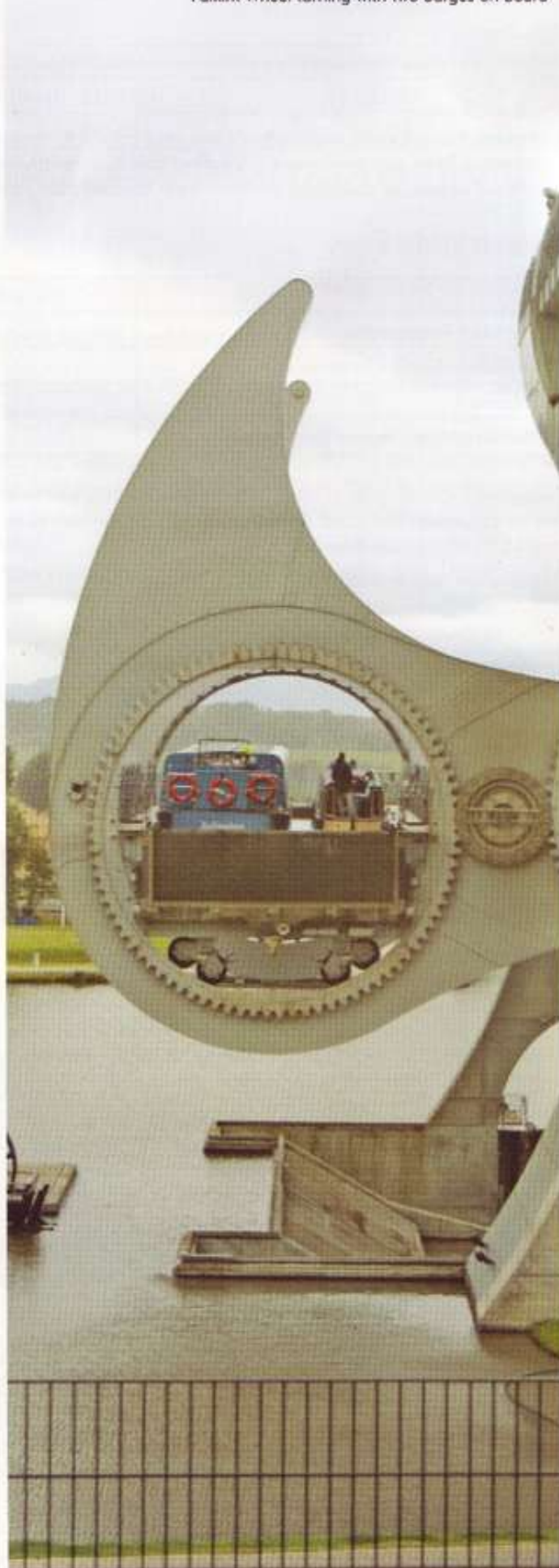
Falkirk Wheel turning with two barges on board
